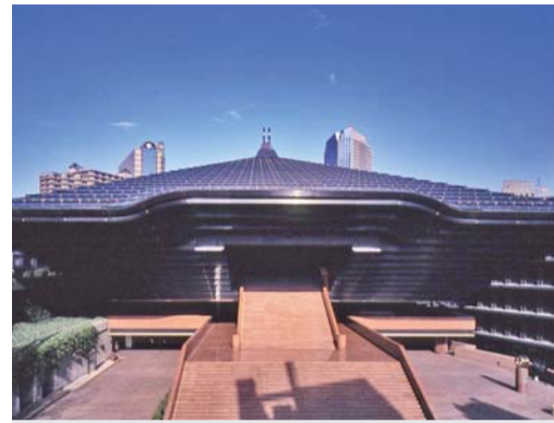
The electrochemically colored shingles on Tokyo's Reiyukai Shakeden Temple have not faded since they were installed in 1975. Photo courtesy of JSSA (building) and Catherine Houska (detail)
