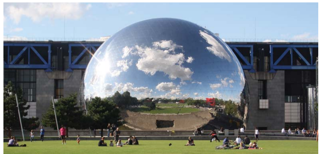
Located in the Parisian museum known as the City of Science and Industry, La Géode is an Omnimax theatre, covered by a geodesic dome with almost 6500 mirror-finished Type 316 panels. Photo courtesy of ParisSharing
