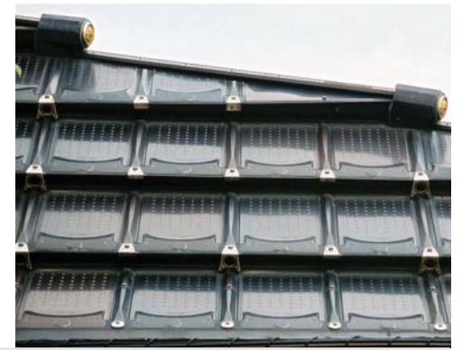
The electrochemically colored shingles on Tokyo's Reiyukai Shakeden Temple have not faded since they were installed in 1975. Photo courtesy of JSSA (building) and Catherine Houska (detail)
