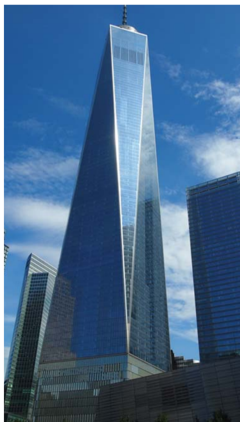
At 541 meters, One World Trade Center is the tallest building in the western hemisphere. Type 316L supports the podium's glass fins, accents the glass tower's façade corners and forms the 6-ton spire.
