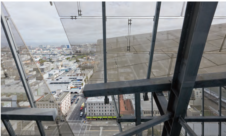
The perforated Type 316 sun screen panels can be individually rotated with changing sun position to vary the level of shading. © Iwan Baan
