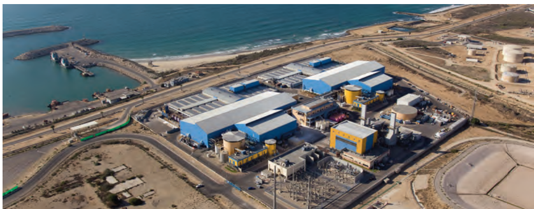
Figure 2: The Ashkelon RO desalination plant in Israel. © IDE Technologies
