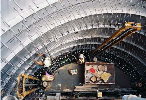
Figure 5: Shear connectors on the inside of a tower segment
