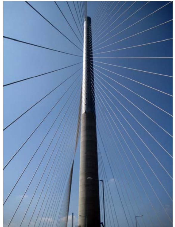
Figure 2: Mono tower and stay cables
