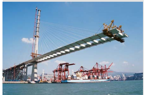
Figure 4: Bridge under construction
