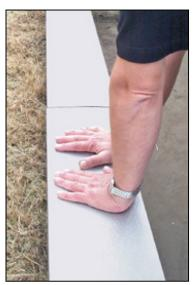
Adhesive bonding is a practical solution in building applications, when stainless steel has to be fastened to masonry or natural stone
