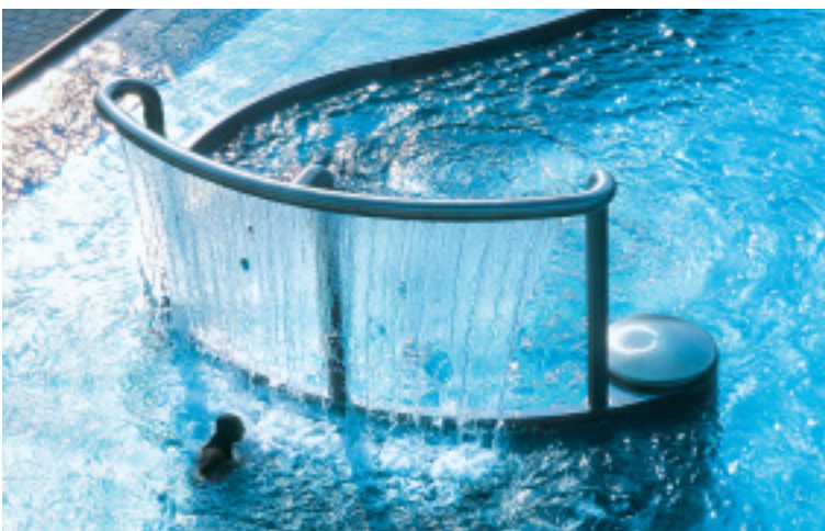
High air and water temperatures, coupled with constant water movement, raise the chloride content close to the pool, even in outdoor facilities.
