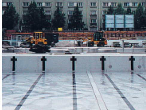
The black lane markings on the floor of the swimmers' pool were applied to the panels electrolytically.
