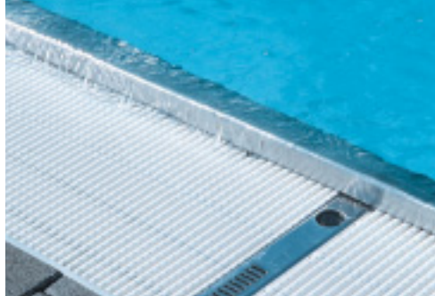
Overflow gutters transport the pool water back to the collector tank.
