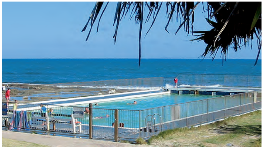
Figure A Stainless steel is used regularly for coastal applications. If properly selected, it can remain attractive and structurally sound in this corrosive environment. (Photo Courtesy of Australian Stainless Steel Development Association)
