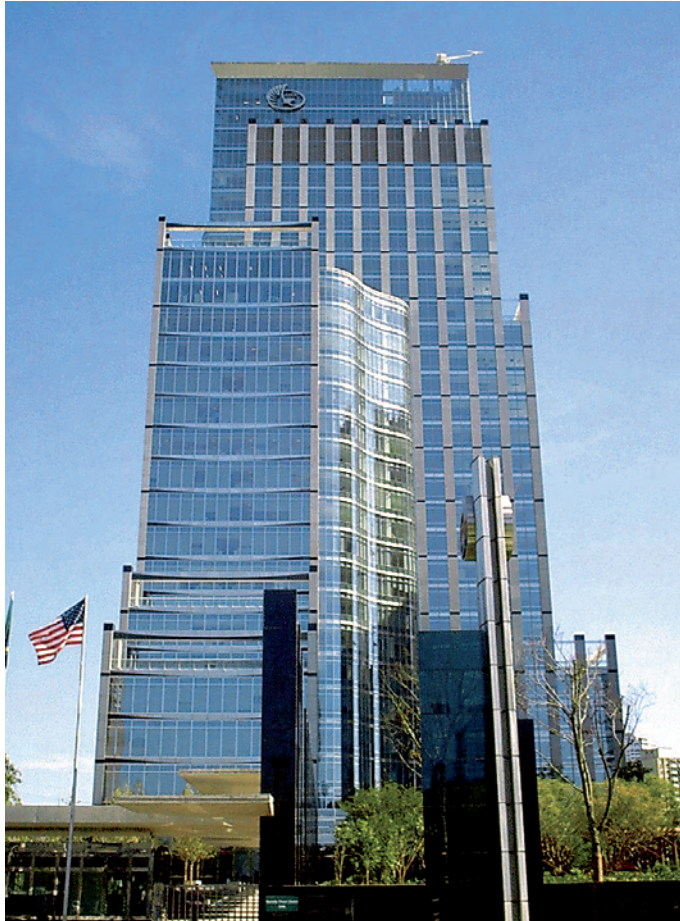
Figure A Careful stainless steel selection, design and maintenance ensure that the exterior will remain beautiful over time. (Photo Courtesy of Núcleo Inox)
