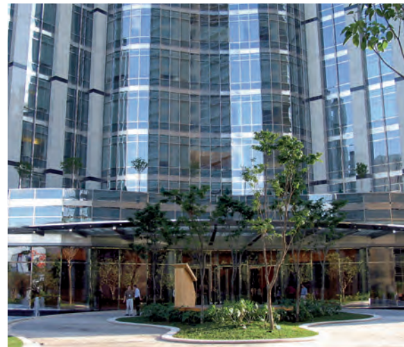
Figure B All three stainless steel finishes can be seen around the building's park-like entrance. (Photo Courtesy of Núcleo Inox)
