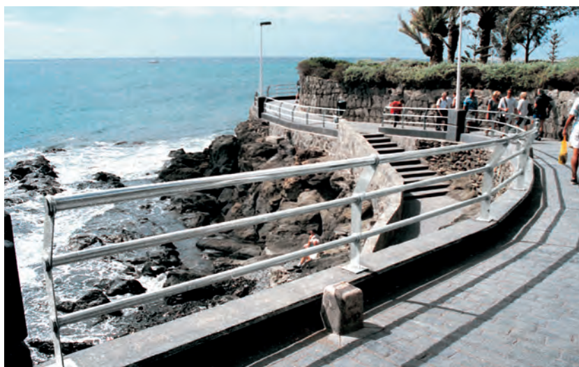
Figure A These 2205 stainless steel railings are exposed to salt spray and occasional splashing. They are in the town of San Augustin in the Canary Islands. There has been no corrosion staining despite exposure to sea spray. (Photo Courtesy of Outokumpu)
