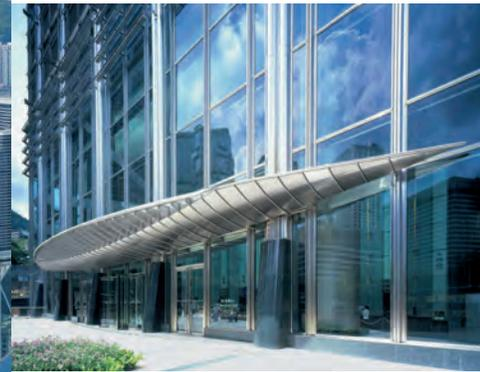
**Figure A and B** Cheung Kong Center is the high-rise building in the foreground of Figure A. The entrance and other details are visible in Figure B. Type 316 stainless steel with smooth surface finishes was an excellent choice because it is exposed to pollution and coastal salt. Window washing tracks were built into the building for easy cleaning. As shown in Figure A, it is in close proximity to the harbor. (Photos Courtesy of Outokumpu)
