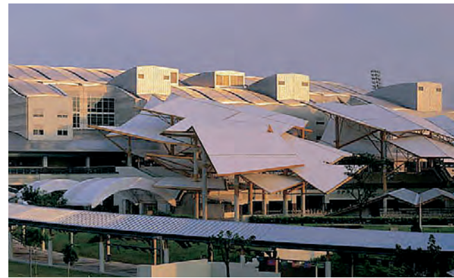
Figure A The Type 316 stainless steel roof of the Singapore Turf Club's grandstand and covered walkway appears to change color during the day. It reflects sunrises, sunsets, blue skies, and clouds. (Photo Courtesy of Ewing Cole, Photographer: Erhard Pfeiffer)
