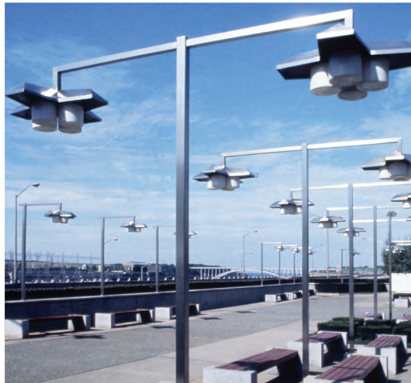
Figure A Boldly exposed Type 316 stainless steel light poles with a smooth finish provide good performance in most coastal applications. (Photo Courtesy of AISI)
