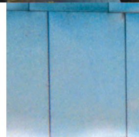
Figure A (above) Type 316 stainless steel with a smooth surface finish and a design that encourages rain cleaning was the right choice for the Weisman Art Museum. Although it is beside a busy road where deicing salt is used, there is no corrosion. The color of the building changes constantly as it reflects the surrounding environment.
