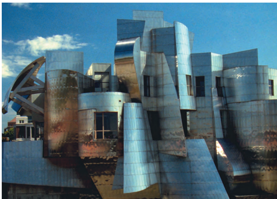
Figure A (above) Type 316 stainless steel with a smooth surface finish and a design that encourages rain cleaning was the right choice for the Weisman Art Museum. Although it is beside a busy road where deicing salt is used, there is no corrosion. The color of the building changes constantly as it reflects the surrounding environment.
