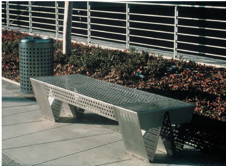
Figure A Specification of Type 316 stainless steel, a smooth finish and a design that takes advantage of rain washing keep this bench and handrail beautiful. (Photo Courtesy of Paul Pittsford)
