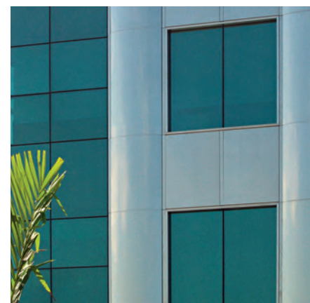
Figure B Close-up of the building exterior. Photo Courtesy of Núcleo Inox
