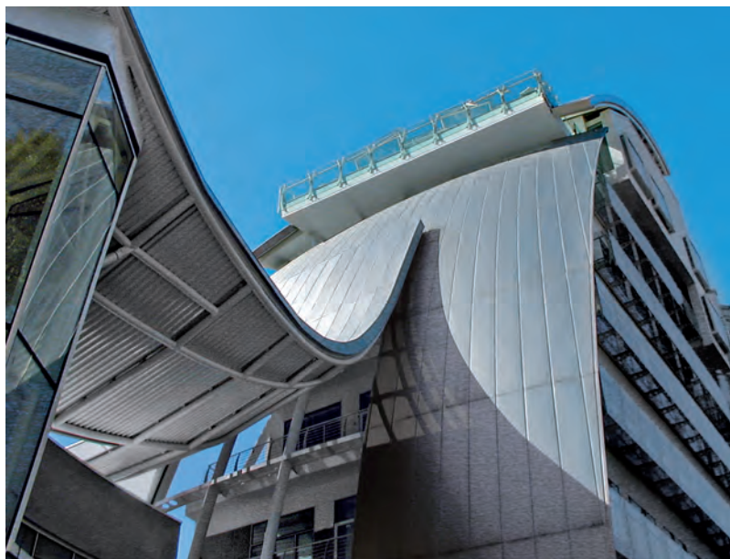
Figure A The new office building has a perforated, seven-story Type 316L stainless steel "sail" that also serves as a sunscreen. Photo courtesy of Centro Inox.
