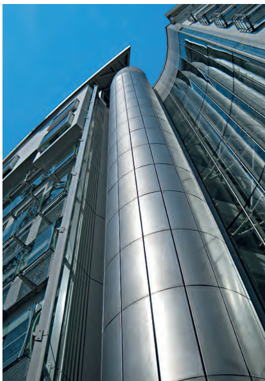
Figure B Type 316L stainless steel covers the columnar elevator shaft at the point where the buildings were joined. Photo courtesy of Centro Inox.
