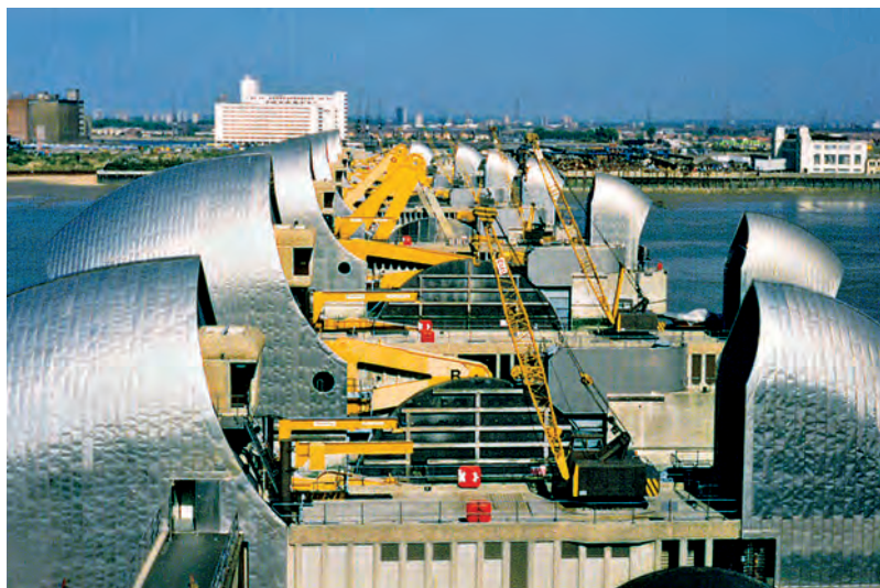
Figure A The Thames Barrier’s gleaming Type 316 stainless steel shortly after it opened in 1982. (Photo courtesy of the Nickel Institute)
