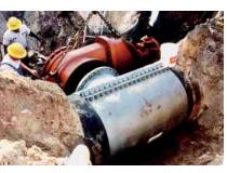
**Stainless Steel Tapping Sleeve** Large diameter tapping sleeve (Photo Courtesy of JCM Industries)
