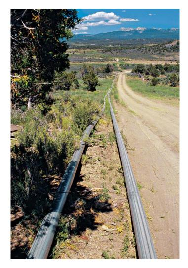
**Stainless Steel Water Pipe** Above ground application (Photo Courtesy of the Nickel Institute)
