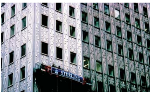
Figure 1. In 1995, the exterior of New York's 150 East 42nd Street (formerly Socony Mobil Building) was cleaned for the first time in 40 years, removing dirt and hydrocarbon accumulations. Photo courtesy of ATI Allegheny Ludlum
