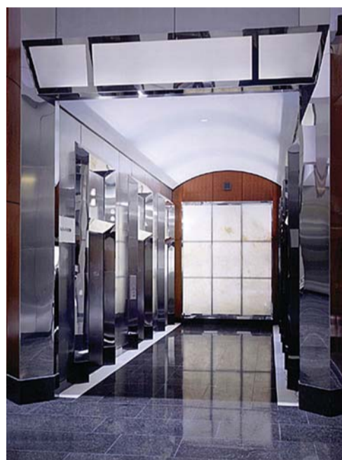
Figure 6. After 50 years of oil and wax 'cleaning,' the stainless steel in this lobby was dark from dirt and grime accumulation and had some scratching (top). The panels were taken down, cleaned with dishwashing detergent, refinished with non-metallic abrasive pads, reshaped and reused in the new design (bottom). Any unused metal was recycled after the reshaping. Bottom photo courtesy of IKM
