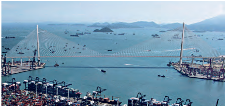
Stonecutters Bridge, Hong Kong. © Ove Arup & Partners
