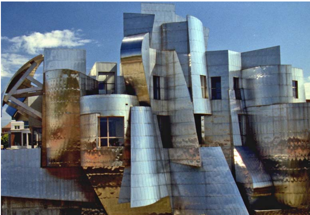
Figure 1: The Frederick R Weisman Art Museum has a smooth, fine No. 4 finish on its Type 316 stainless steel exterior and is easily rain-washed. It has performed well despite significant annual deicing salt exposure. No corrosion staining was evident on the exterior although there was some dirt accumulation.
