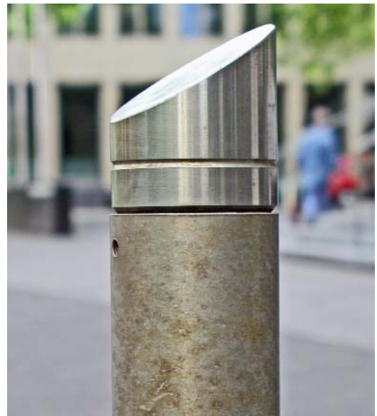
Figure 10: Type 316 stainless steel bollard adjoining a Düsseldorf, Germany roadway. Image courtesy of the International Molybdenum Association, Nicole Kinsman photographer
