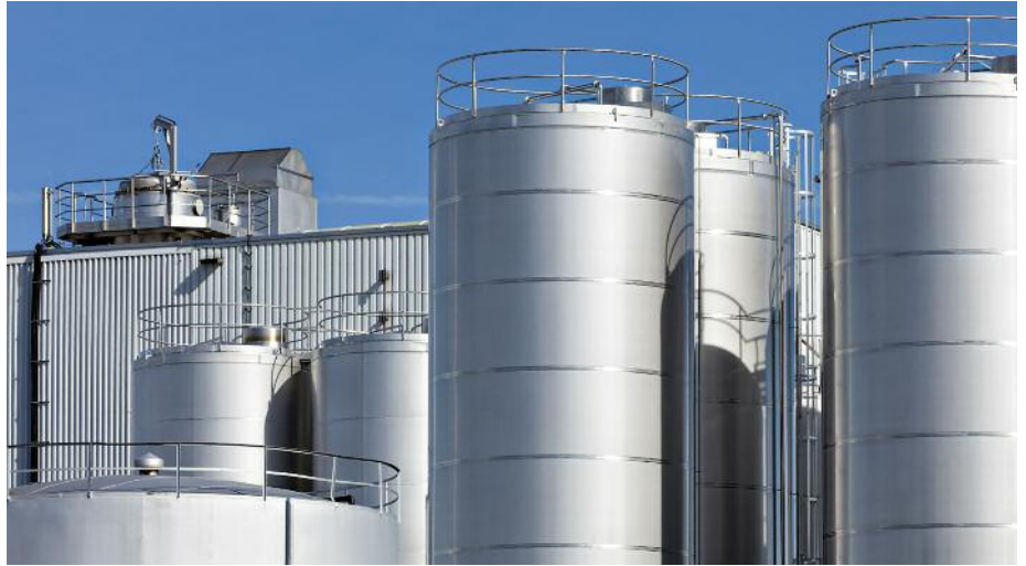
乳品厂的不锈钢焊接储罐。© iStock.com/Bim
