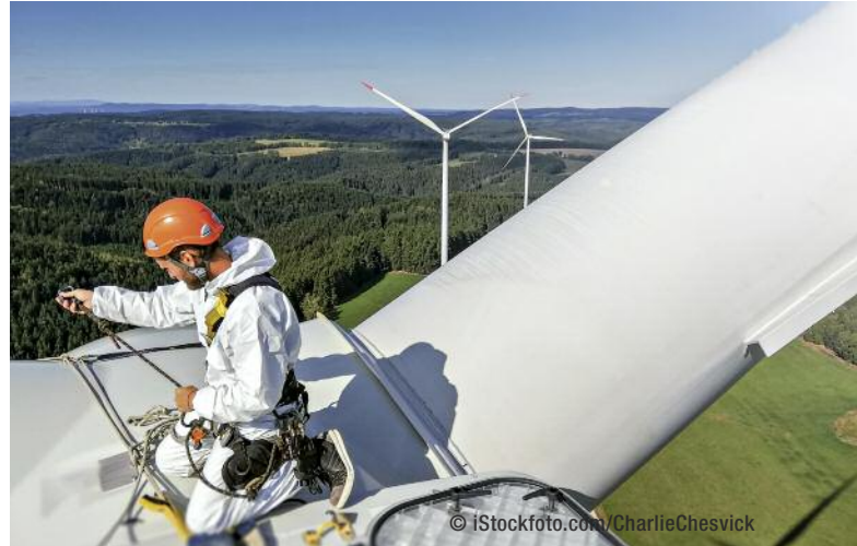
➤ Wind turbines are difficult to access for maintenance and repair as the nacelle sits high above ground. Better materials can reduce the need for costly interventions.
