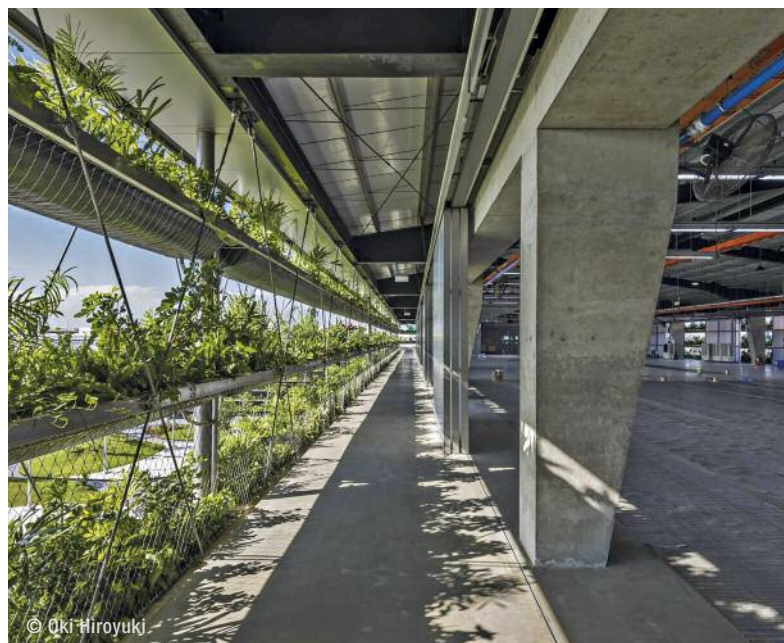
➤ Sliding polycarbonate dividers, fixed in front of the factory's concrete support columns, can be closed in extreme weather.
