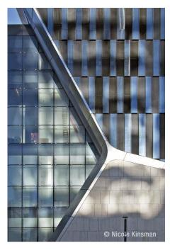
Massive stainless steel panels clad part of the base of 15 Hudson Yards.
