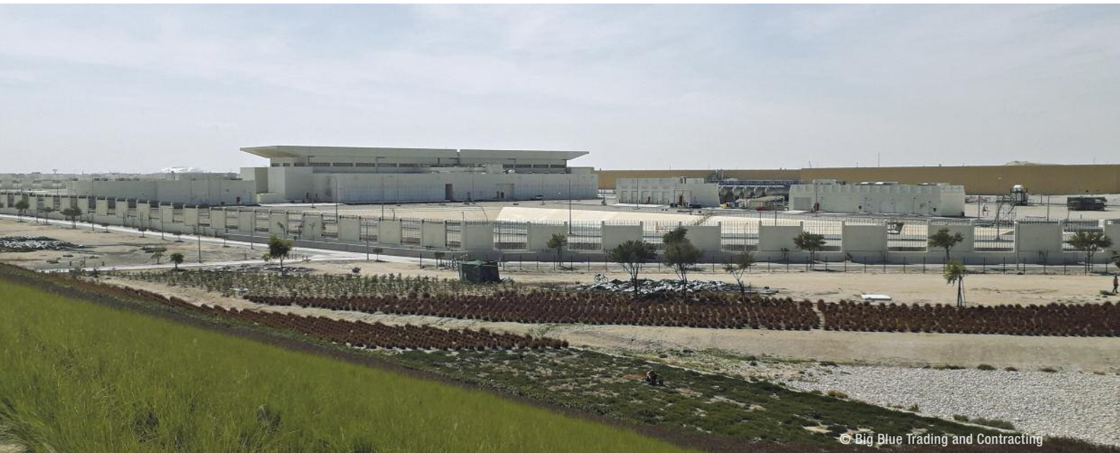
➤ One of the mega reservoirs at a distance. They will be filled with drinking water beginning in 2020.
