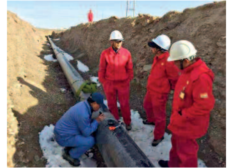
Workers inspecting the new pipeline. © Cheng Xingbao
