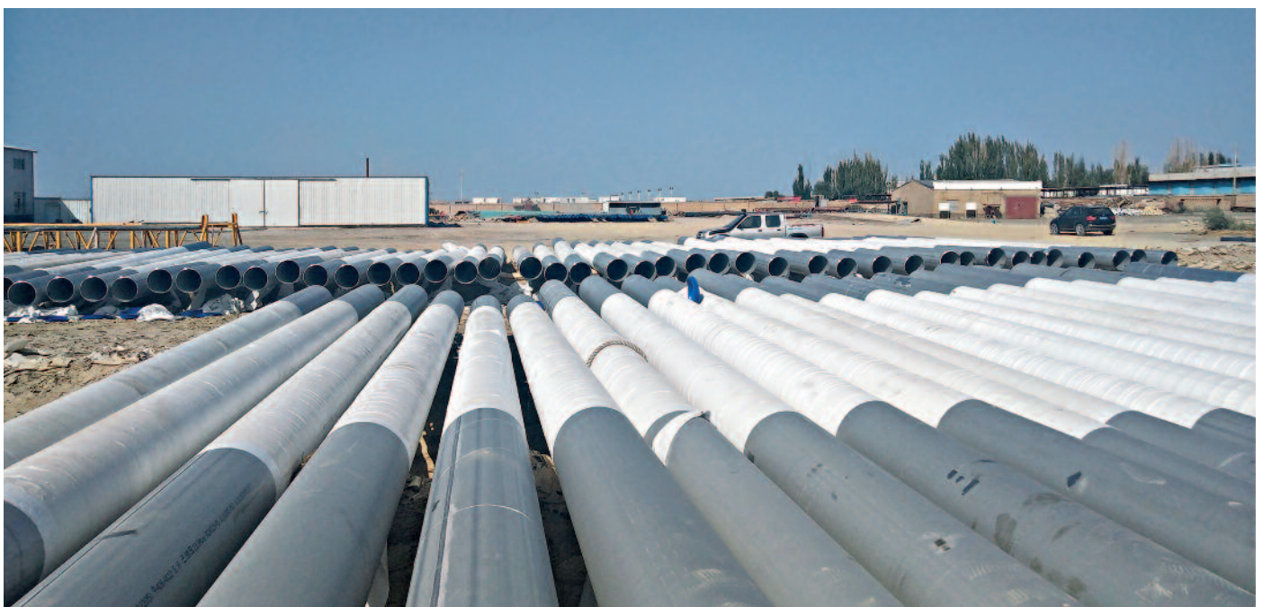
Duplex stainless steel pipes awaiting installation in the field. © Wang Qinghai
