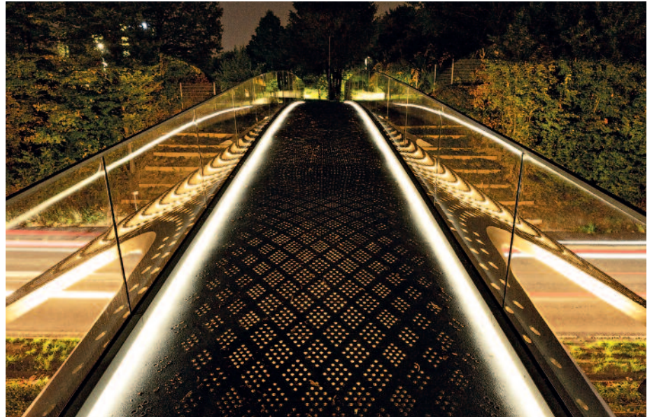
At night, LED lights illuminate the bridge on both sides of the walkway and from underneath. © sbp/Andreas Schnubel
