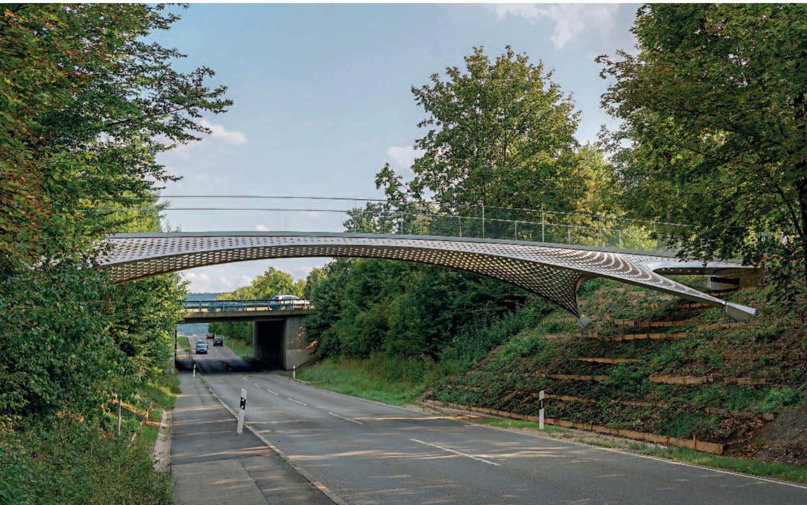
Due to the optimized design, the bridge is so light, it appears to float over the road. © sbp/Andreas Schnubel
