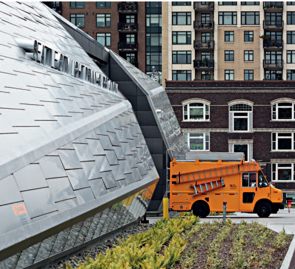
Type 316 stainless steel panels offer a modern aesthetic to an often overlooked public utility. © Samuel Sproule
