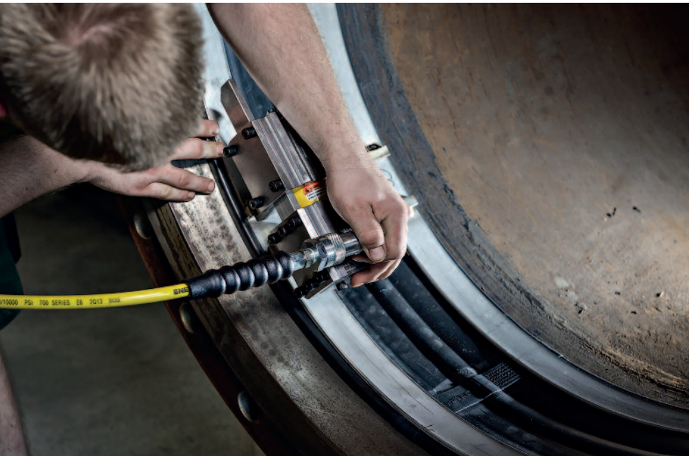
Installation of the internal pipe sealing system. © AMEX
