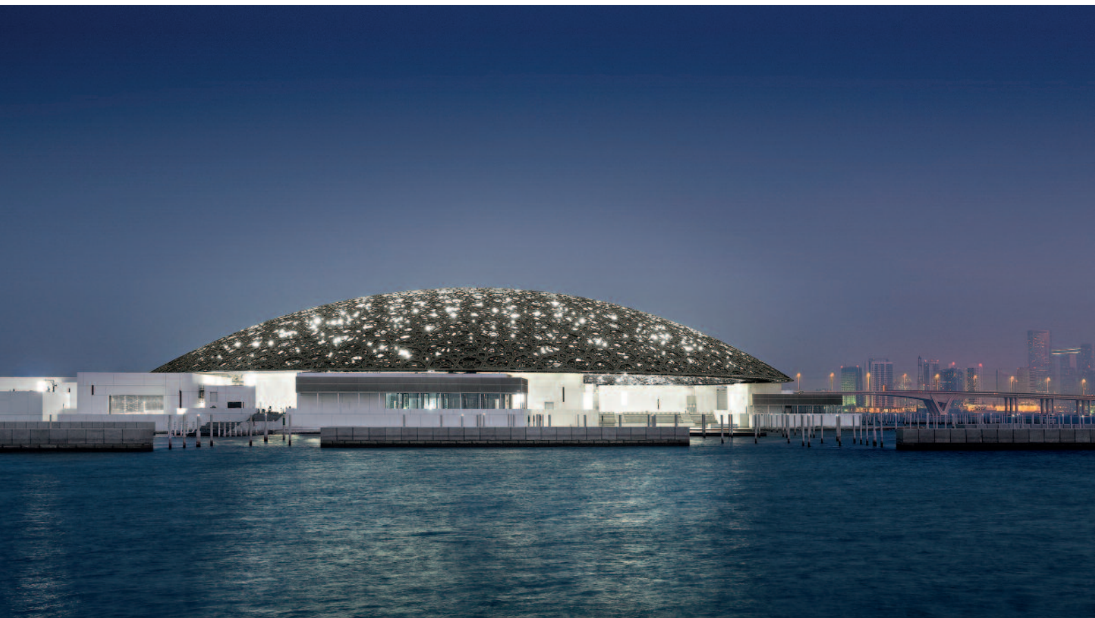
At night, the dome sparkles from the inside. The stainless steel reinforced concrete walls in the foreground protect the museum from the sea. © Louvre Abu Dhabi – photography Mohamed Somji – Architect Jean Nouvel
