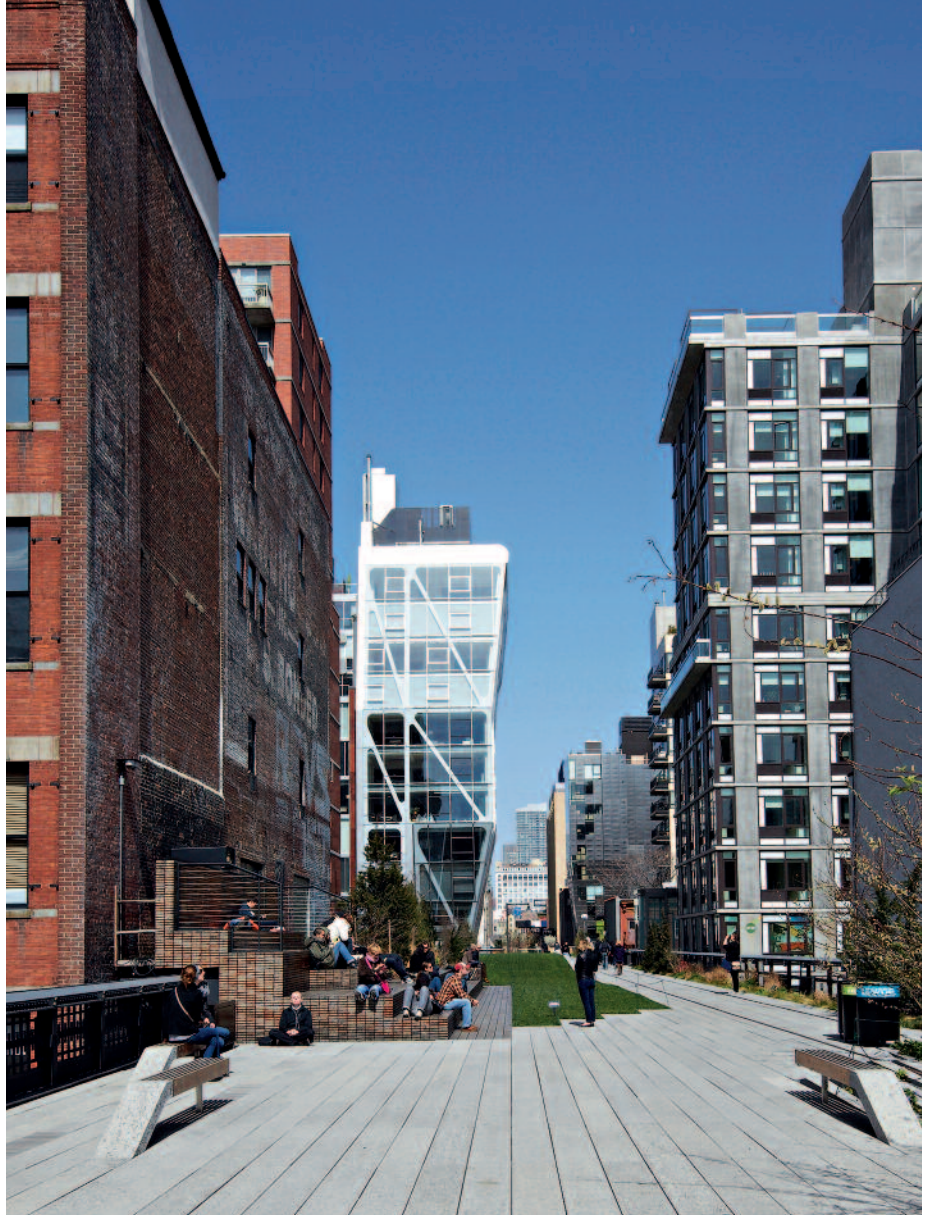
The elevated High Line park is embedded in the neighborhood. Some stretches are flanked by buildings on either side and new ones are added every year. © Jakob Rope Systems
