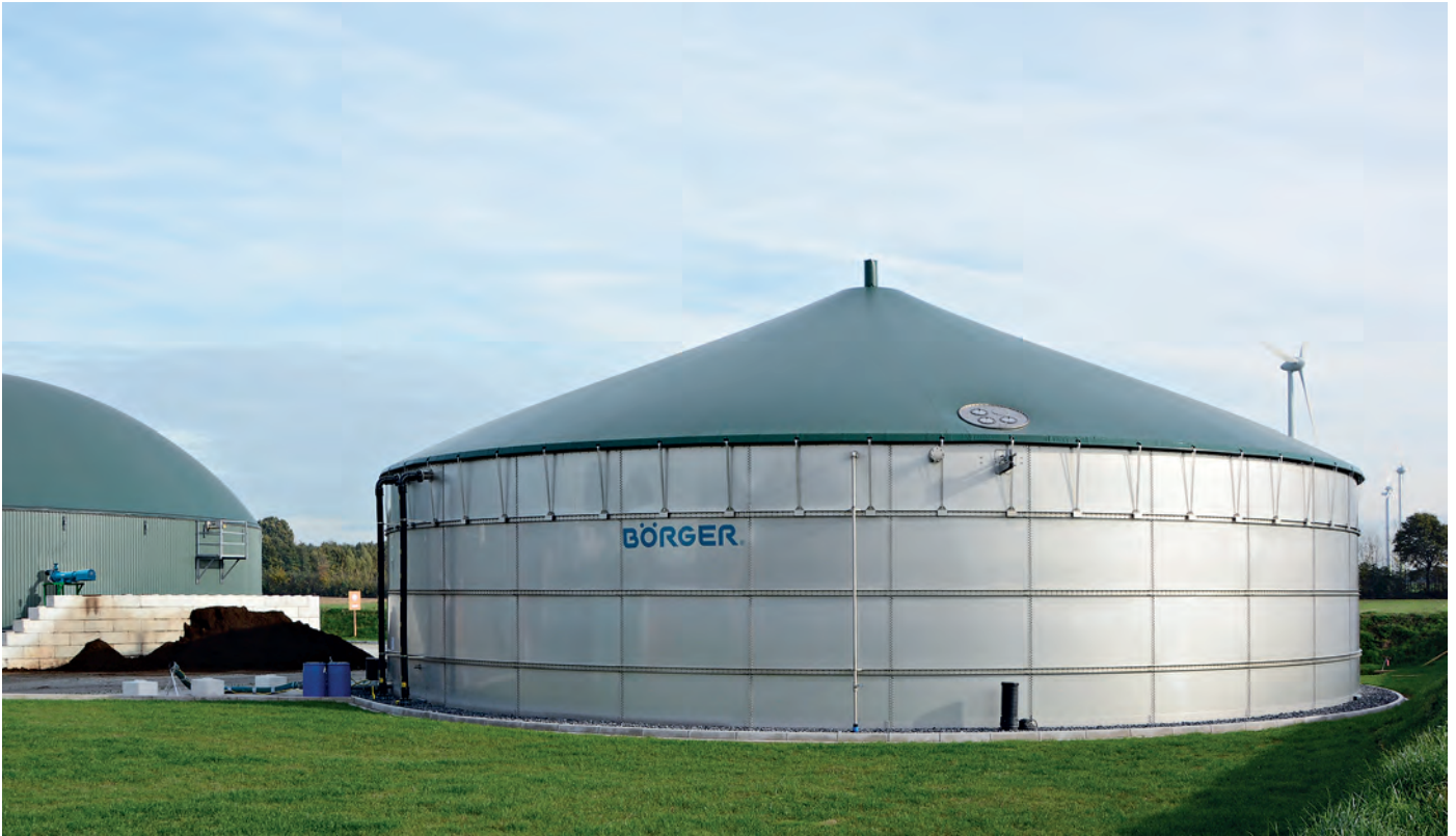
A biogas tank made of LDX 2404 in Germany. © Börger GmbH
