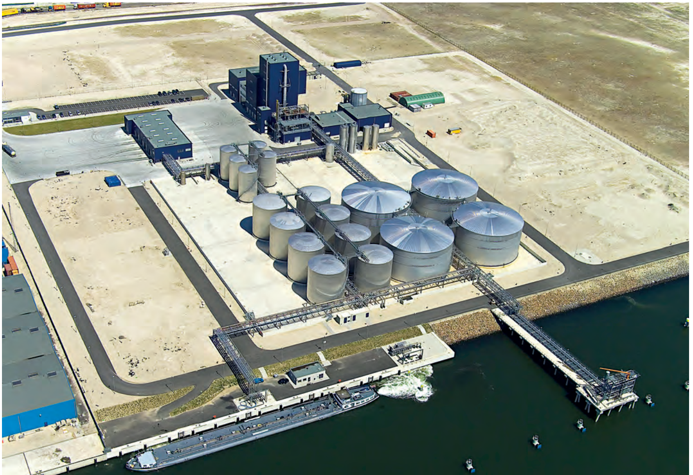
Palm oil storage tanks in Holland made of LDX 2101® stainless steel. © Lodders Crokiaan
