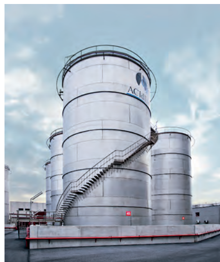
2304 duplex stainless steel tanks at the tank terminal in Bilbao, Spain. © Outokumpu/Acedika
