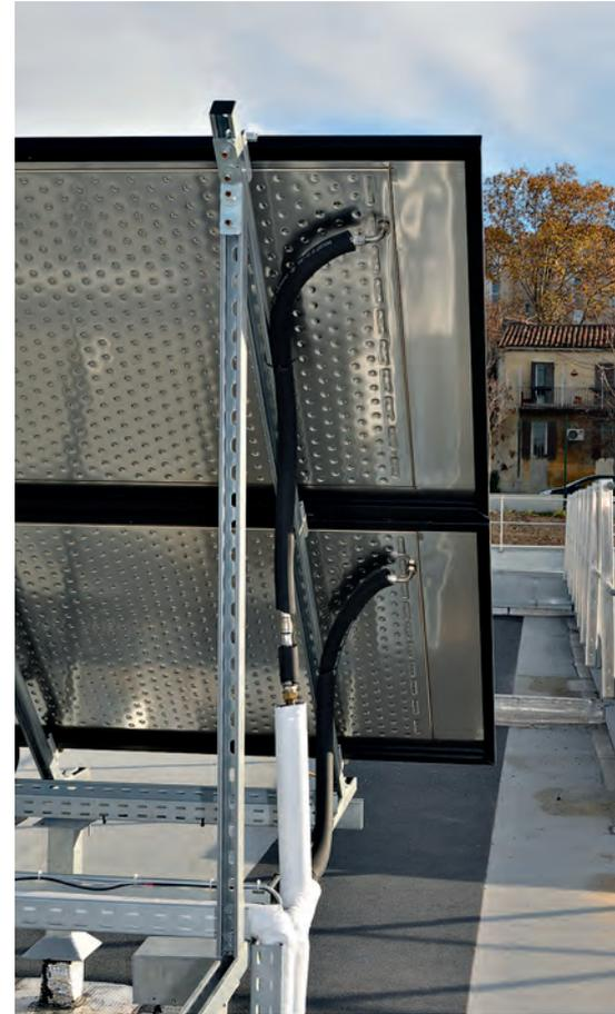
Coolant flows inside the stainless steel heat exchanger just beneath the solar panel, stabilizing its temperature and transferring its heat through another heat exchanger to produce domestic hot water. © DualSun
