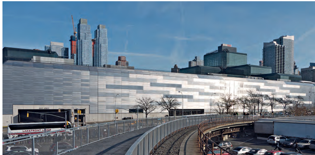
Three different Type 316 finishes add visual interest to Javits Convention Center. © Nicole Kinsman
