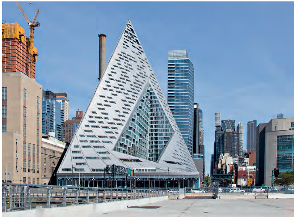
The innovative VIA 57 WEST was designed to be the world's most sustainable residential building. © Contrarian Metal Resources/Gabby Pignanelli
