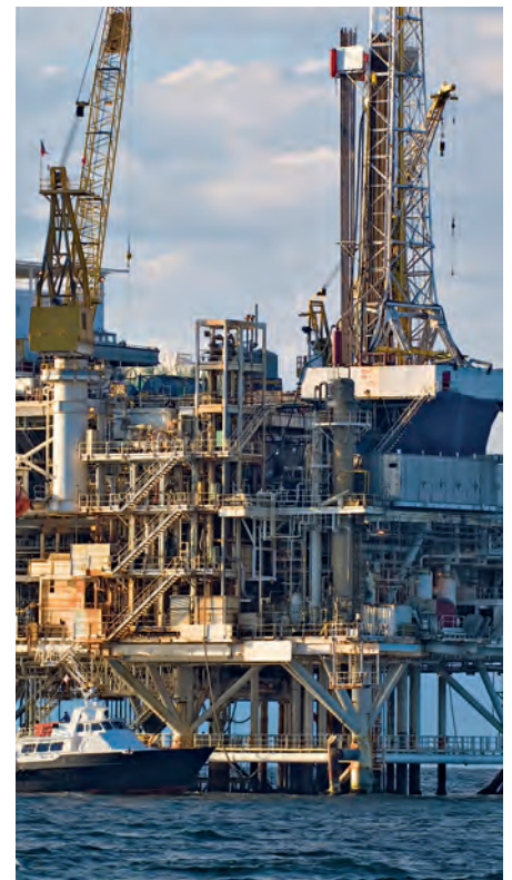
Offshore platforms constitute a harsh environment, requiring high performance alloys for many applications. © iStockphoto/Arthurpreston
