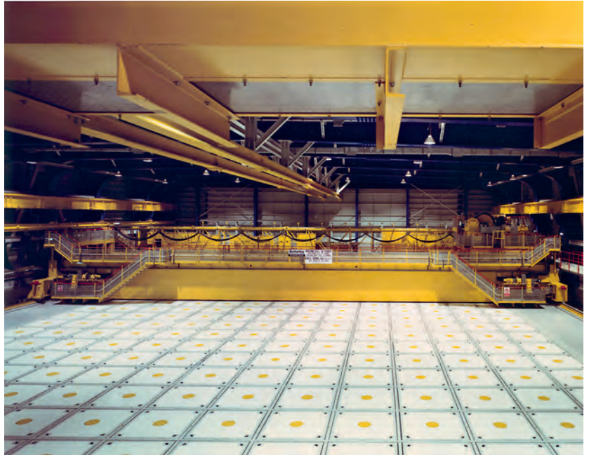
Intermediate level waste drums at Sellafield made from Type 316L stainless steel. The drums are filled with waste and stored in stacks (one stack of ten drums under each white square with the yellow dot) in the Encapsulated Product Store at Sellafield, prior to final geological disposal. © Sellafield Ltd
