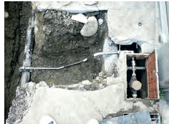
Installation of corrugated Type 316 stainless steel service pipe in Tokyo. © Tokyo Waterworks
