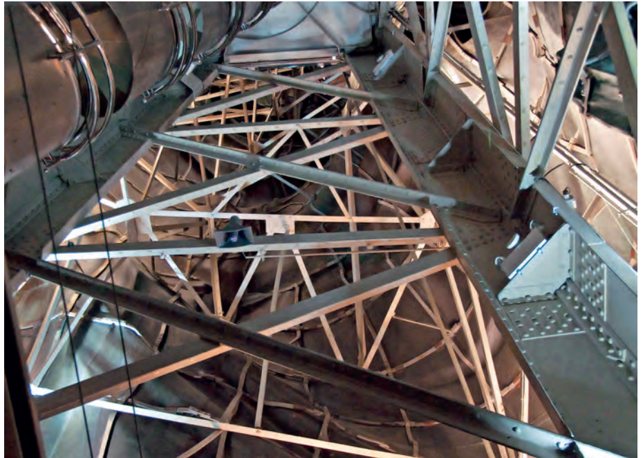
Looking up through the central pylon the intricate detail of the unique structure built to support the statue's façade can be seen. © Mike Renlund
