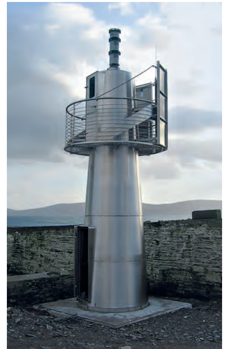
The finished Roancarrigmore lighthouse, a new high-technology replacement for its venerable predecessor. © Commissioners of Irish Lights
