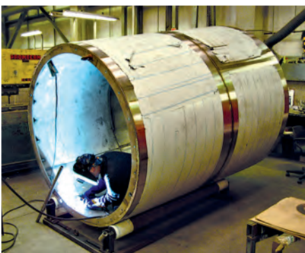
Fabricating a shell section of the Roanarrigmore lighthouse tower. © Commissioners of Irish Lights
