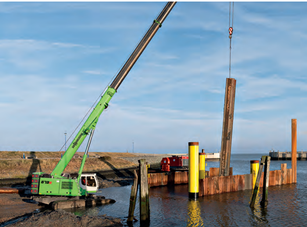
Crawler cranes are the "heavy lifters" of the crane family, and are widely used for construction projects. © SENNEBOGEN Maschinenfabrik GmbH
