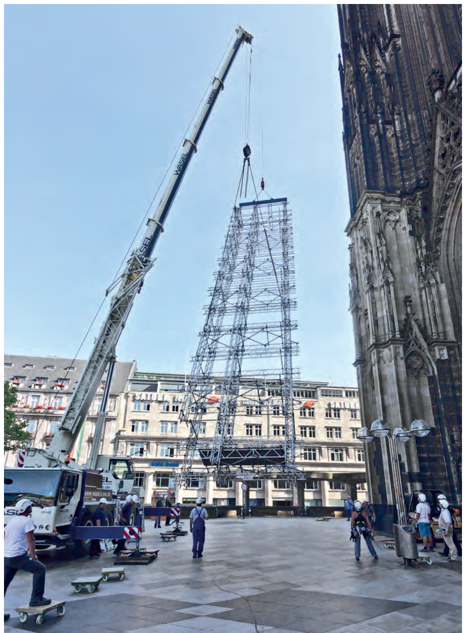
The Cologne Cathedral’s scaffolding is carefully lowered to the ground during its removal following restoration work. © Raimond Spekking/CC BY-SA 3.0 (via Wikimedia Commons)
