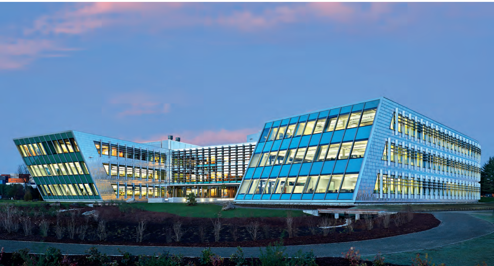
The stainless steel shingles on the façade shimmer in many shades like fish scales. © Benjamin Benschneider/OTTO
