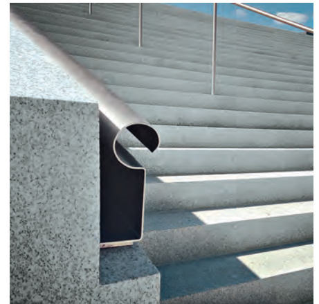
The custom made duplex handrails blend in with the granite. © Diane Bondareff
