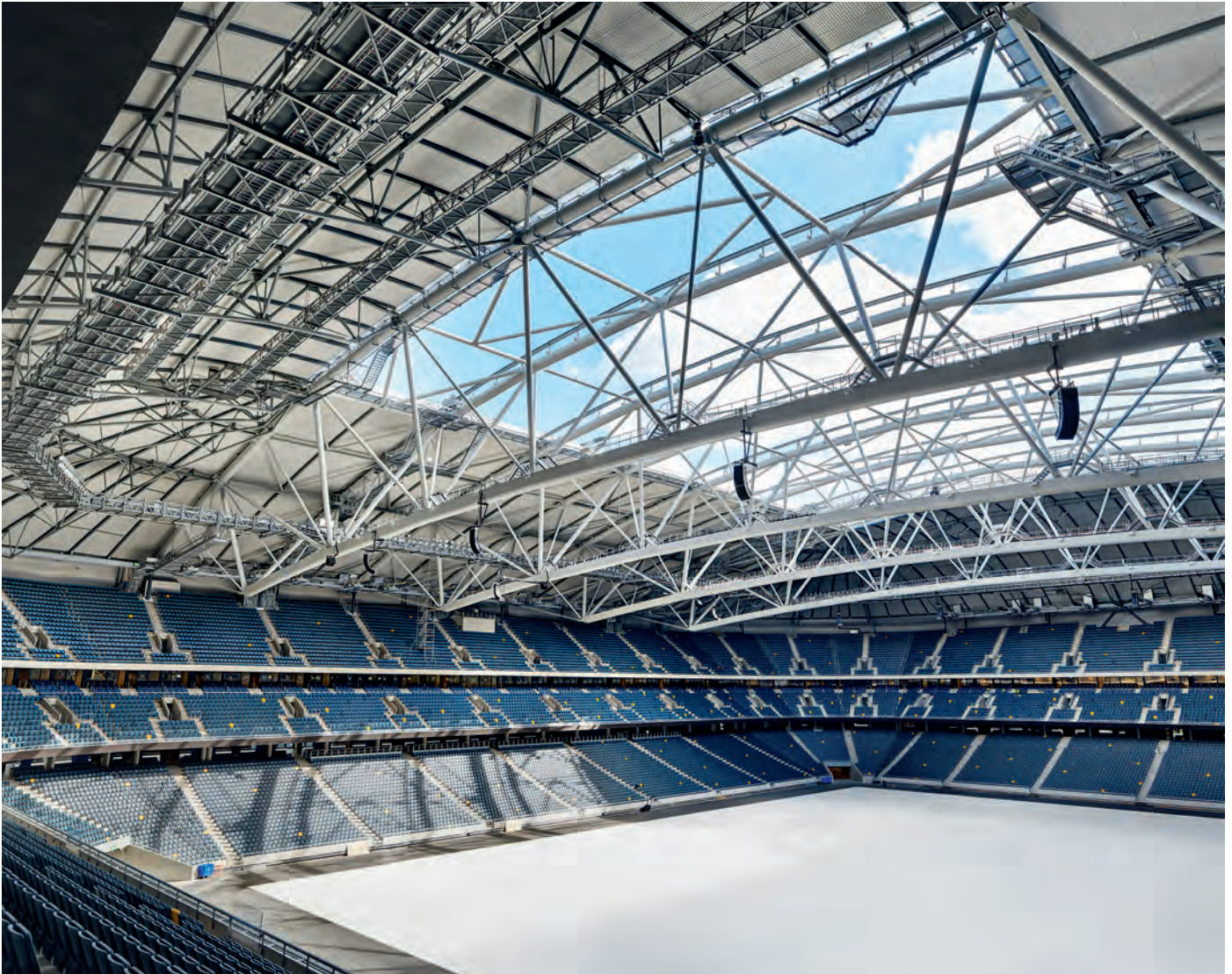
High-strength steel trusses supporting the retractable roof. © Sweden Arena Management
