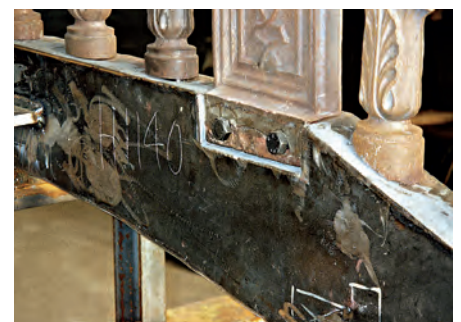
Stainless steel reinforcing plates were welded to the inside faces in a workshop (below). From the outside, the restored bridge looks like the original, the repairs are invisible. © (below) Insula spa, municipal agency for the urban maintenance of Venice.
