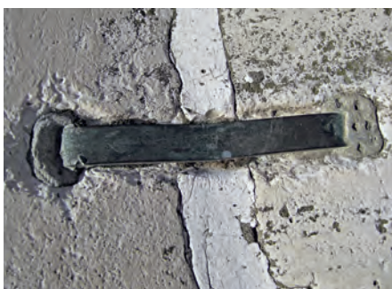
The white stone caps of the brick walls are secured with metal brackets. The original copper or iron brackets (left) are now being replaced with Type 316L stainless steel (right).
