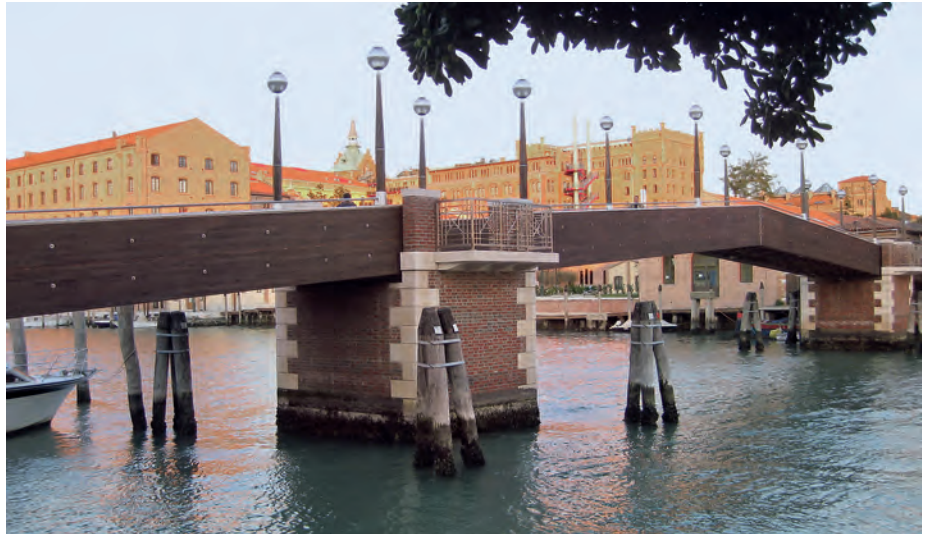
The structure of Ponte dei Lavraneri is made of 2205 duplex stainless steel. It is the longest bridge in Venice.
