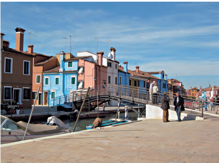
Ponte delle Capuccine on Burano is built from Type 316L and painted black to blend with the historic environment.
