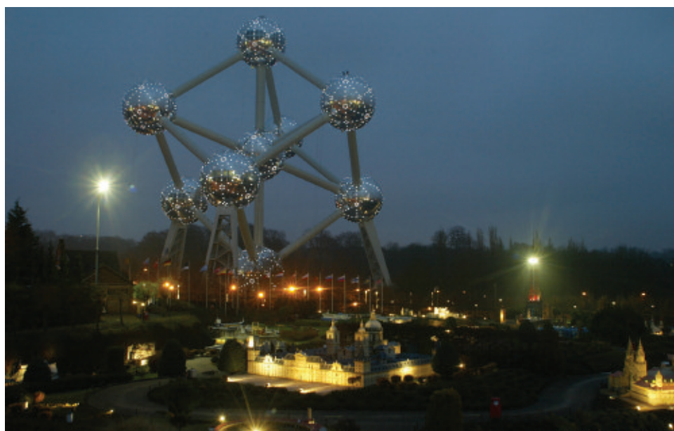
Figure 4: The Atomium in Brussels is clad with Type 316 molybdenum grade stainless steel (Courtesy of Nickel Institute)
