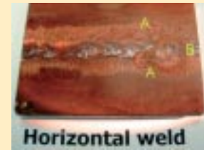
Figure 1. View of the horizontal weld piece, showing pitting in the base plate (A) and the weld (B). The surface has a brown stain/deposit. The dark color band right next to the weld bead indicates inadequate post-weld cleaning. The coarse grinding marks also lower the pitting resistance.
