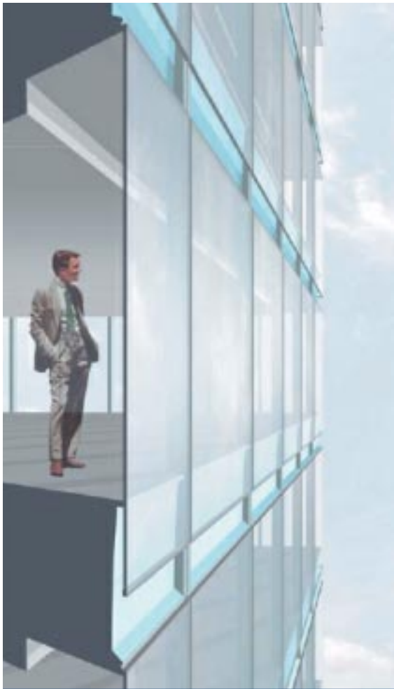
A rendering of the spandrel and blue-colored Type 316 panels that will be used between each floor in the office tower.
