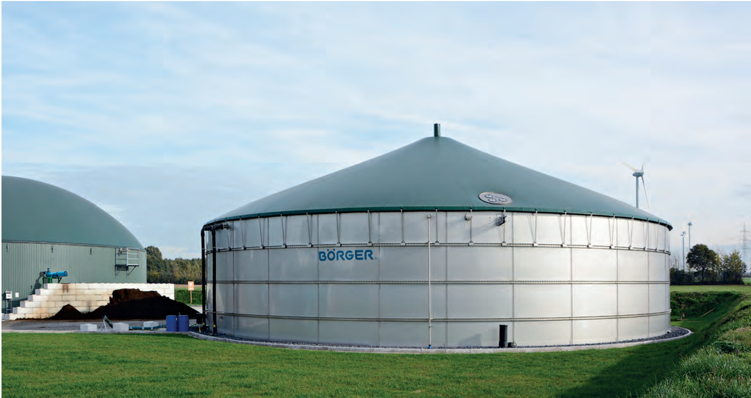
A biogas tank made of LDX 2404 in Germany. © Börger GmbH
