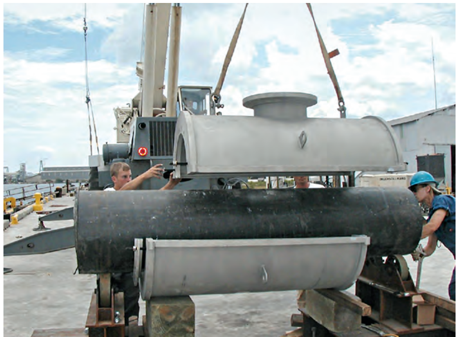
“Mock” installation of a custom-fabricated Type 316 stainless steel repair sleeve. The technicians are practicing the underwater installation on a piece of pipe in the dry. © Charleston Commissioners of Public Works
