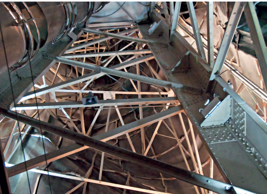
Looking up through the central pylon the intricate detail of the unique structure built to support the statue's façade can be seen. © Mike Renlund
